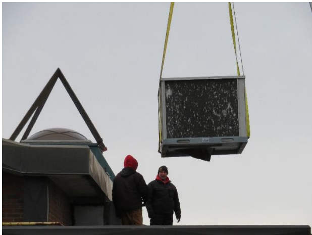
Property committee oversee the installation of new air conditioner
