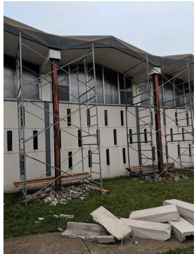
The property Committee is taking on the reconstruction of the posts in auditorium area.
